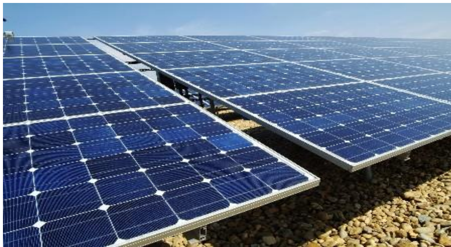
Gambar 2.4. Panel surya Polykristal
