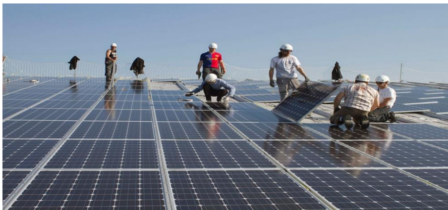
Gambar 2.3. Panel surya Monokristal
